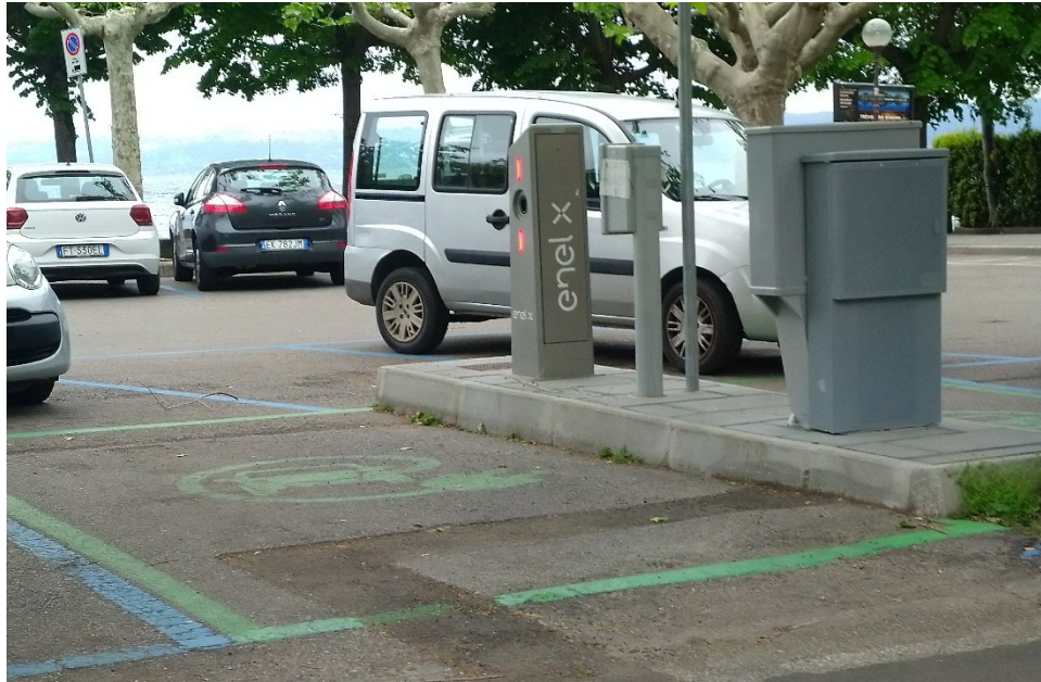
Figure 8. Municipality of Trevignano Romano, charging station for electrically powered vehicles - EnelX Project [Source: Photo by Authors].
