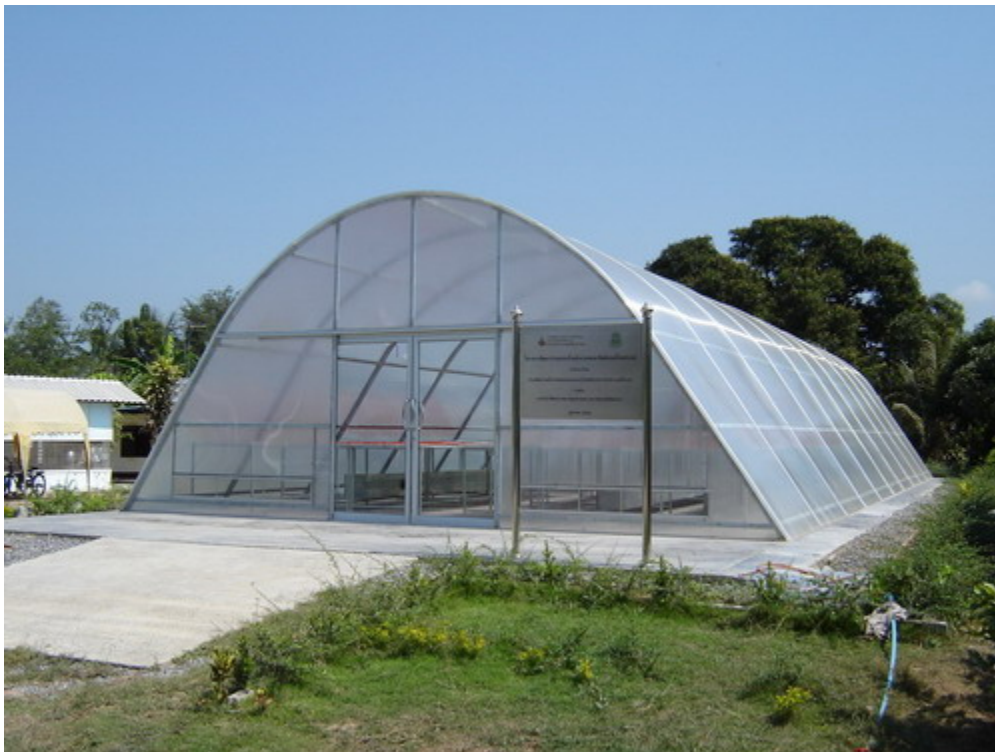
Figure 1. Pictorial view of the large-scale solar greenhouse dryer with LPG burner
