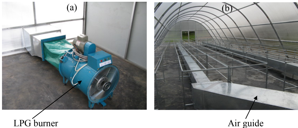
Figure 2. A pictorial view of the burner (a) and air guides (b)
