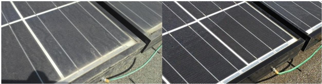
Figure 8. Cleaning of the modules of the GO' grid-connected PV system. Source: The authors.
