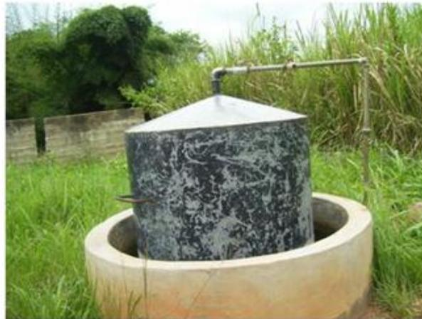
Figure 9. A water-jacket floating-drum plant at an abandoned slaughterhouse at Tepa in Ahafo-Ano north district of Ghana, September, 2008
