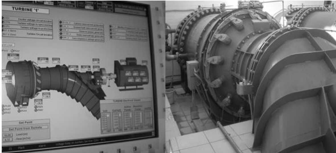
Figure 6. Small Hydropower Scheme with one S-Kaplan turbine recovering the wasted energy applying the P.D.P. in the Kithairon site of the Athenian aqueduct.
