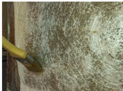
7- Putting the resin mixture on fibers
