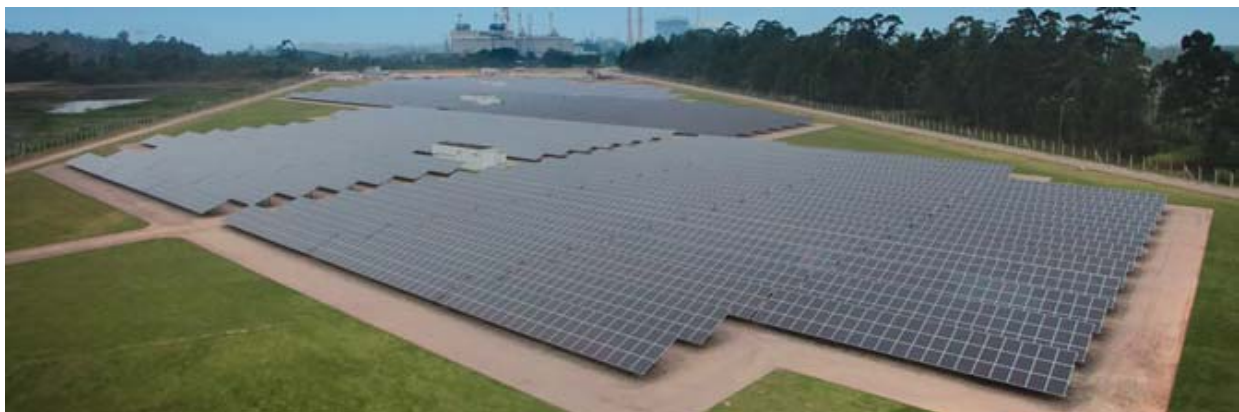
Figure 5. Cidade Azul photovoltaic power plant's view.
