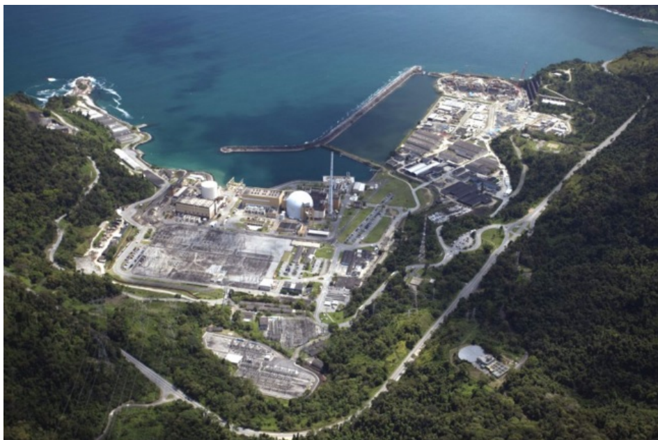
Figure 3. Eletronuclear power plant' view [13].
