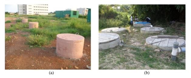
Figure 3. (a) Three 100 m<sup>3</sup> fixed-dome digesters at CUC, Miotso, November, 2008, and (b) Four 10 m<sup>3</sup> Puxin digesters at Hebron Prayer Camp, Hebron, November, 2008
