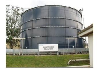
Figure 11. An 800 m<sup>3</sup> UASB bioreactor at Guinness Ghana Breweries Limited, Kumasi, August, 2008
