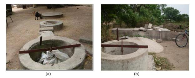
Figure 7. (a) Remains of a Chinese dome at Applonia, February, 2009, and (b) A broken-down Deenbandhu digester at Okushibli; February, 2009
