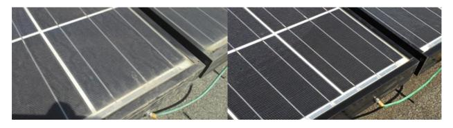
Figure 8. Cleaning of the modules of the GO' grid-connected PV system. Source: The authors.
